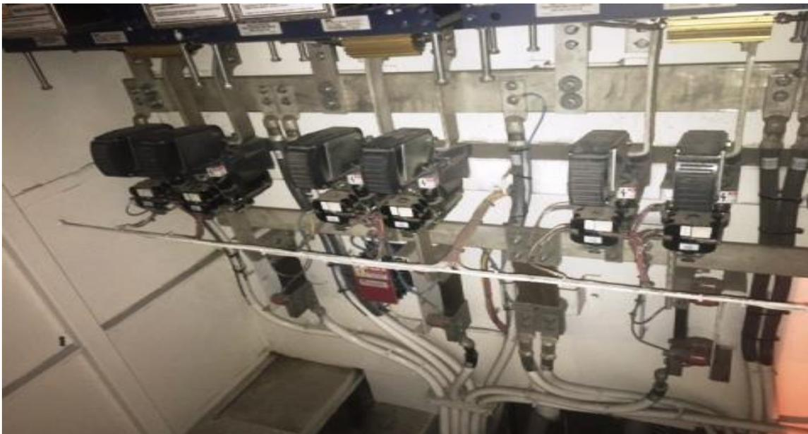
This picture shows the power contactors and associated wiring. Very clean lay out.
