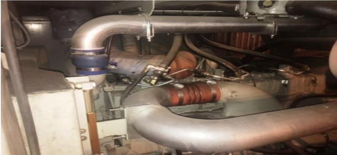
This Cummins engine #1 clean with no oil leaks, well maintained.
