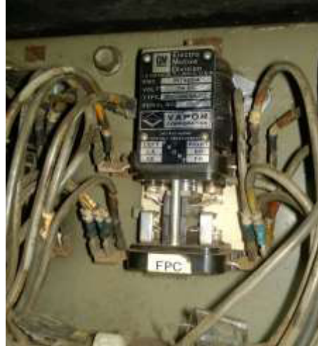
9) FPC relay missing cover.
