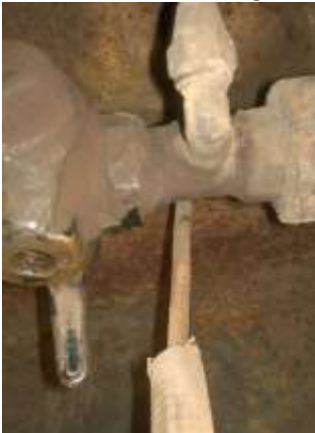
7) Flex conduit for axle generator damaged.
