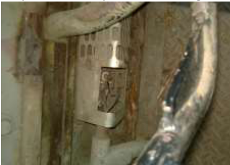
8) Helper's side strip heater missing cover.
