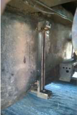
6) Fuel tank sight glass missing sight tube.
