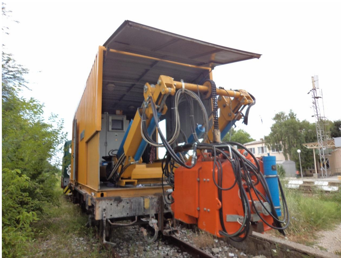
Flash butt rail-welding set.
