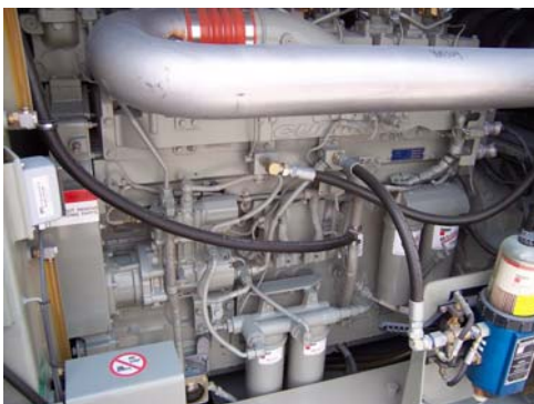
Fig. 7-1 – QSK19 Engine (Installed)
