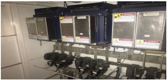
These are the DC choppers located just above the power contactors. Look like new no signs of overheating.
