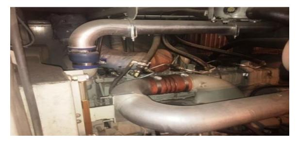
This Cummins engine #1 clean with no oil leaks, well maintained.
