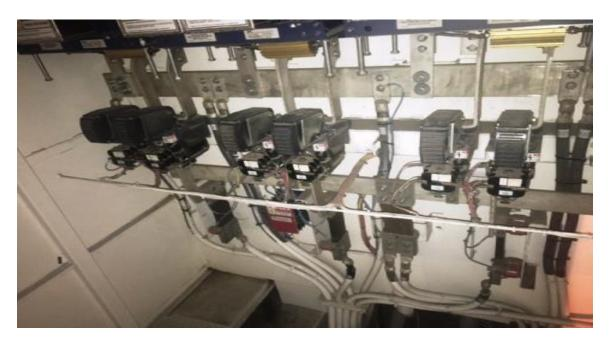
This picture shows the power contactors and associated wiring. Very clean lay out.
