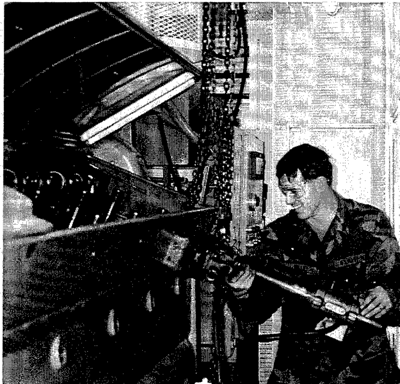
(i) Installing an NG load block.
